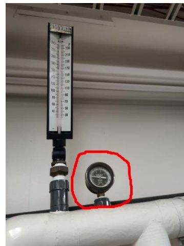
Figure A2. Supply pressure gauge.
